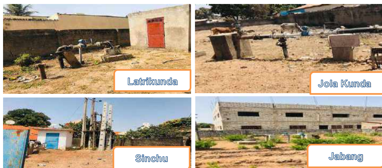
Picture 10: NAWEC boreholes encroached by settlements (Top left PN6(Sinchu), Top right BH12 (Jola Kunda) and BH 18(Latrikunda) all link to the Serekunda WTP and down right is SS6 of Sukuta WTP.
