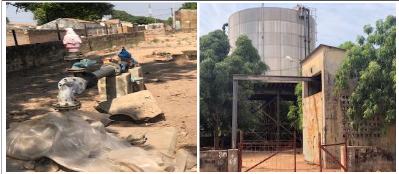
Picture 2: The unprotected water facility at Farafenni (Left) and Mansakonko water facility (right)
